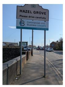
There are 'Welcome to Hazel Grove' signs, mounted on two posts, located in the centre of the footway on both the north and south sides of New Moor Lane. The gap between the two posts supporting the signs is 1250mm, causing unnecessary obstructions.
