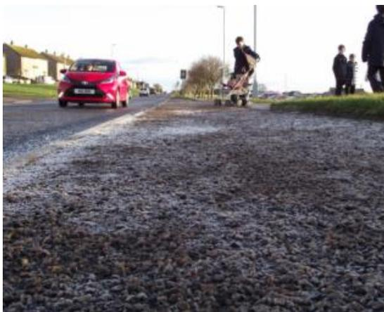
9. DEGRADED FOOTWAY SURFACE ON SOUTH SIDE OF COULARDBANK RD.
