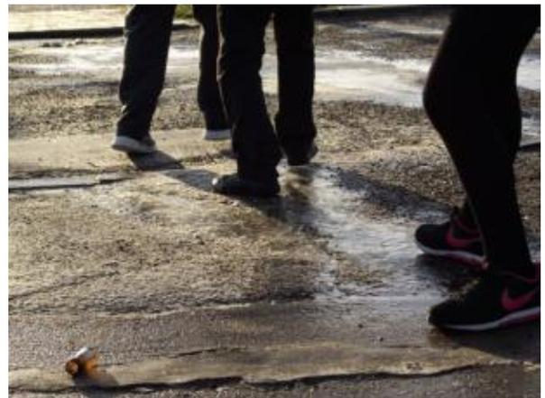
5. FLUSH KERBS AND EDGE MARKERS MISSING. DRAINAGE ISSUES AT CROSSING POINT ON NORTH COVESEA TERRACE
