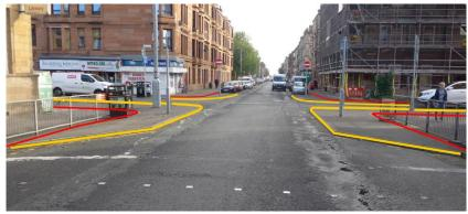
Govanhill also has examples of the alteration of residential junctions to significantly narrow crossing distances, with a raised table proving level access to the carriageway. In the second image below the original positions of the kerbs, and the new kerbs, are highlighted with red and yellow lines.
