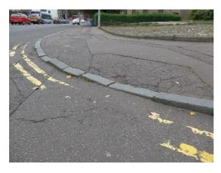
Close up detail from above-right photo, showing low kerb without tactile paving warning.
