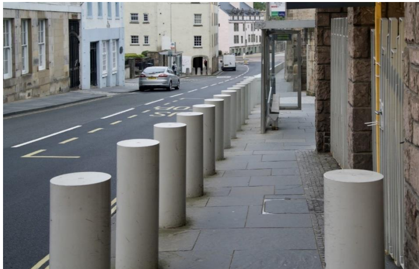
Pinch point at bus stop
