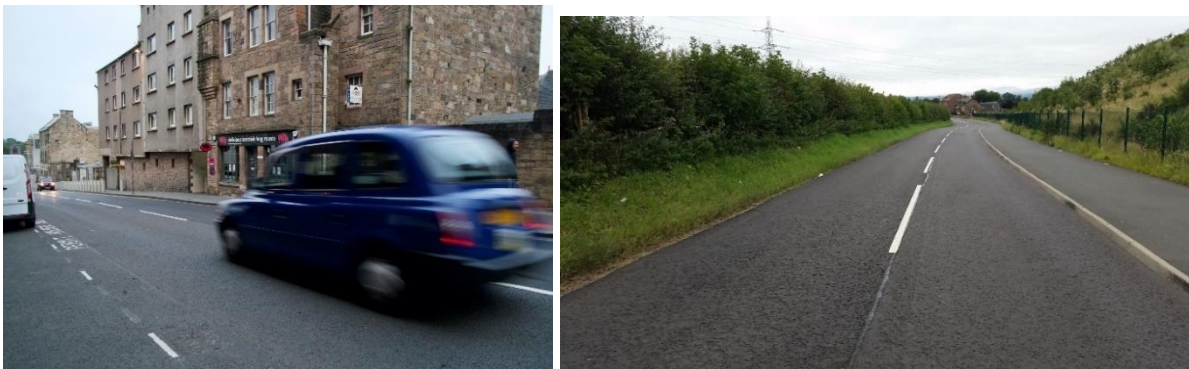
Similar 'warning line' markings used both on Canongate and a fast rural road
