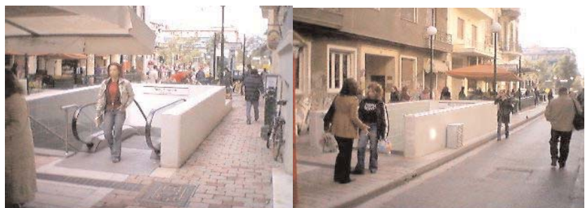
Athens - the metro system was upgraded for the Olympics, including new entrances for stations. Above is the new wider entrance to Victor Square station. But it takes up most of the pavement, leaving just 80 cm to get past. Pedestrians are forced to walk in the road during busy times - an example of how pedestrian facilities can be forgotten when constructing new transport infrastructure. In this example, there would have been room to widen the pavement. How do we avoid similar mistakes being made in the construction projects for the London Olympics?
