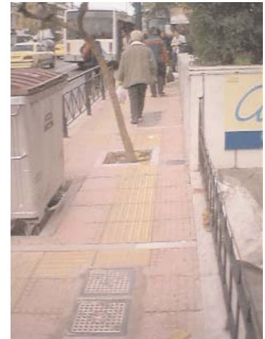
Badly planned pavement improvements for Athens Games - leads disabled people straight into a tree! Opportunities to widen the pavement weren't taken.
