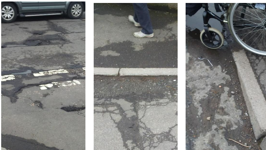
Footway, Carriageway and dropped kerb at Victoria Road
