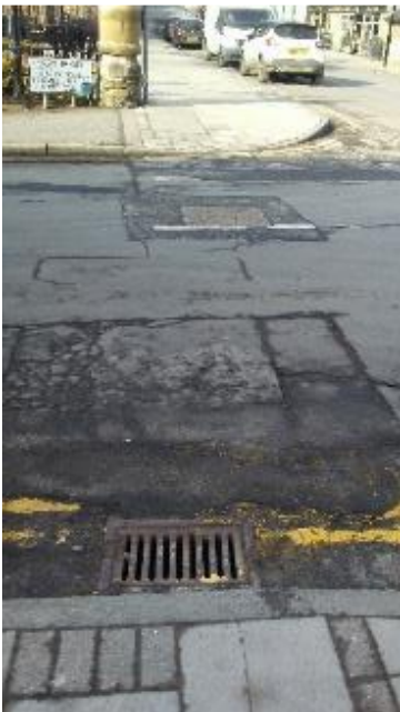
Ferry Road crossing
