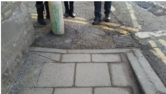
Bollard and low roofline at the Hardware store
