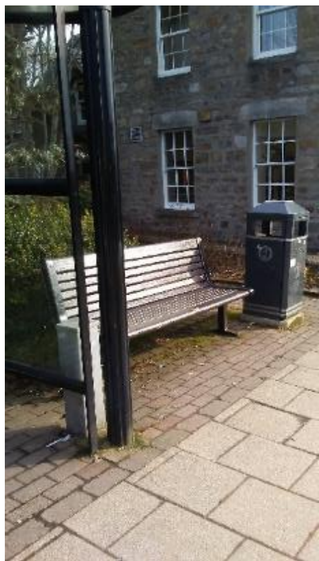
Seating at bus stop
