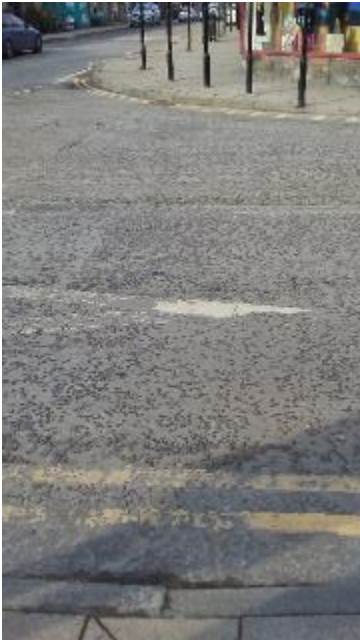
West Moulin Road crossing
