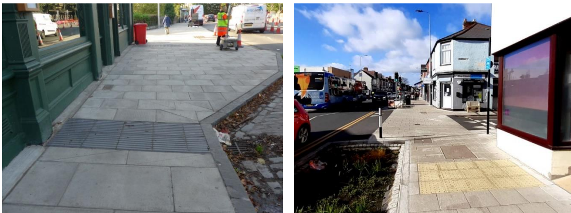
Figure 8: Non-standard layout/style of tactile paving
