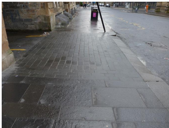
1) Footway appears to continue in an unambiguous way. Drivable space at footway height. Steep access ramp.
