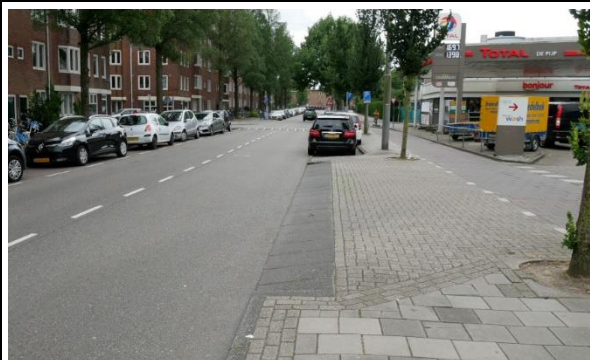
Exit construction (using entrance kerbs) at a Dutch petrol station – part of creating a level footway
