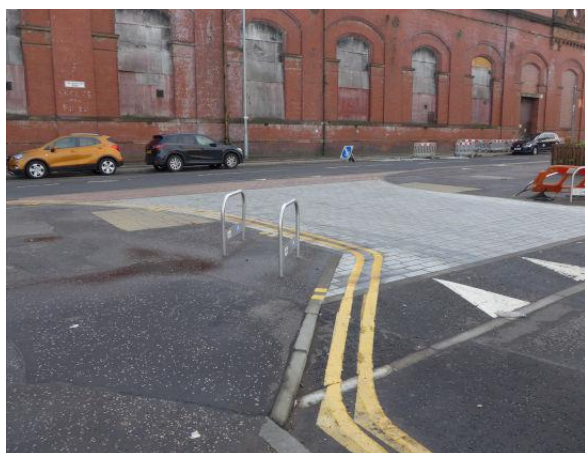
6) Surface implies break in footway. Raised drivable space feels like a speed table.
