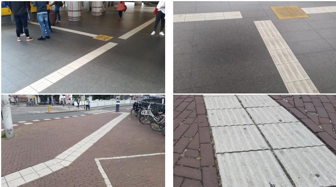
Figure 5: Guide-line paving in the Netherlands
