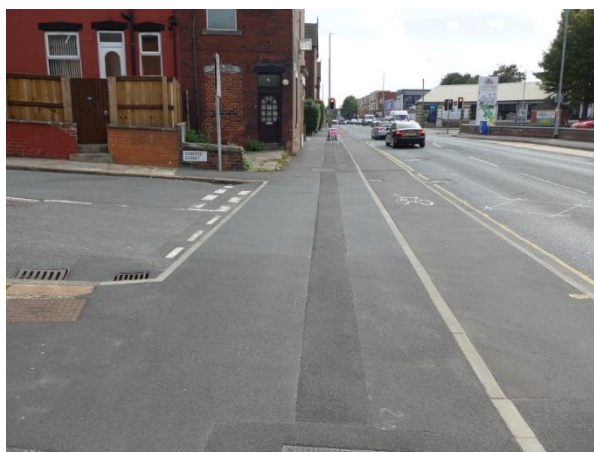
3) Little carriageway-footway contrast. Drivable space at carriage level. Interpreted as continuation of footway?
