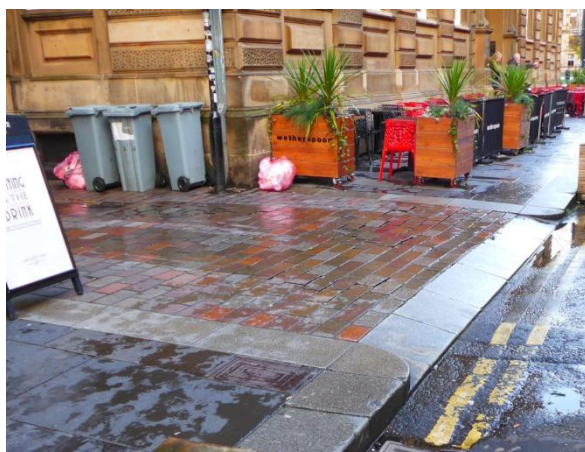
4) Surface implies break in footway. Steep ramp significantly slows vehicles. Drivable space at footway height.
