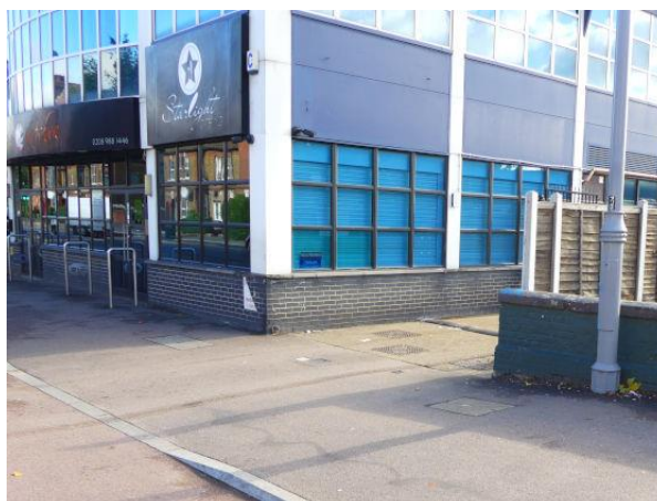
5) Private entrance over footway. Frequent access by large vans. Footway drops to carriage level.
