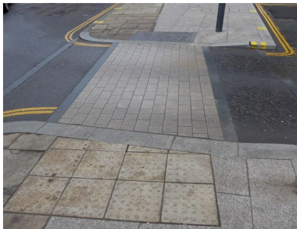
2) Drivable space at carriage height, but significant contrast with carriageway surface and similarity to footway surface.
