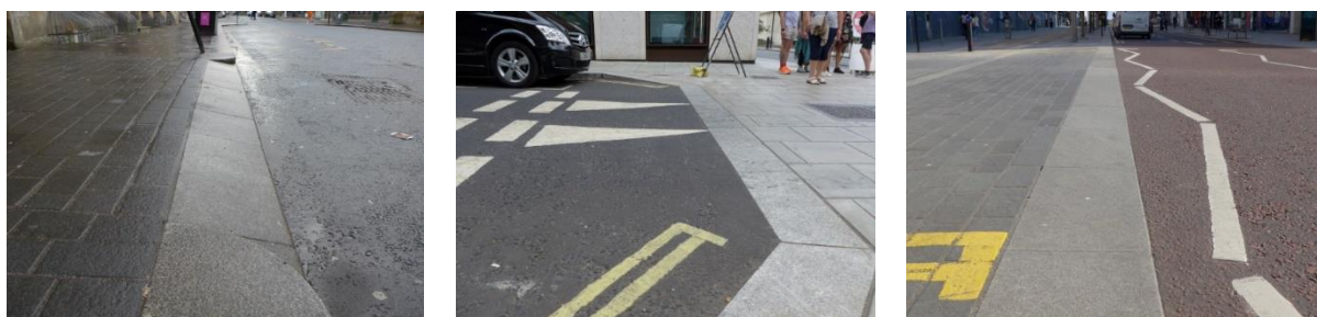
Figure 17: Differing ramp designs (and lack of ramp)
